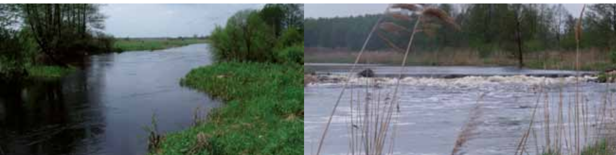
The area of the two already built fault ledges in the Narew riverbed. The image on the left shows fault ledges originally built slightly against the current fault ledge; on the right photo you can see the second fault ledge opened in the spring of 2010.
